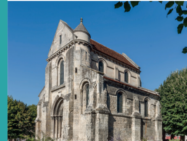
8 Eglise Saint-Pierre St. Peter's Church
